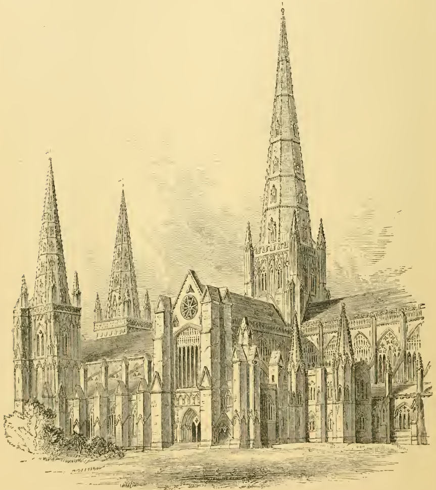
835. View of Lichfield Cathedral. (From Britton's 'Cathedral Antiquities.')
